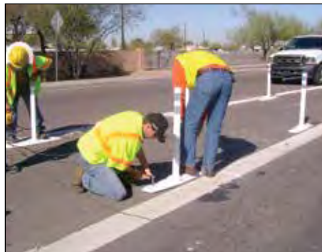
Installing Turnpike Grade Curb
