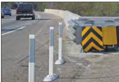
Impact attenuation protection
